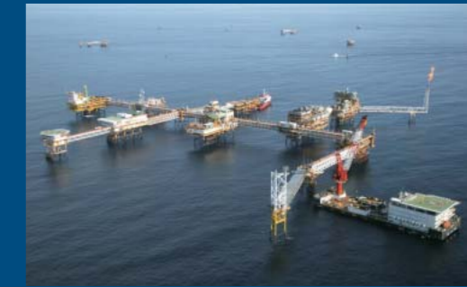
Compressor modules installed on CHAMPION-7 platform, BSP (Brunei)
