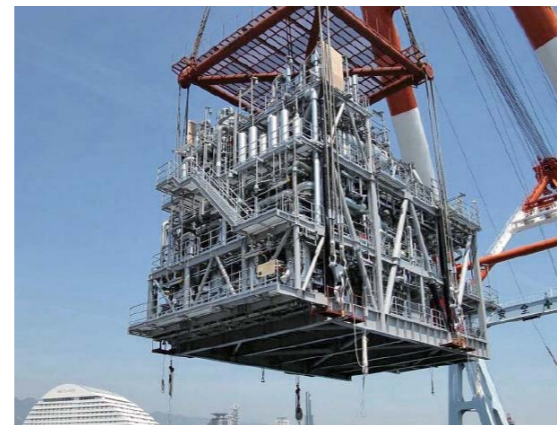
Single lifted Gas Compression Module for KNOC
