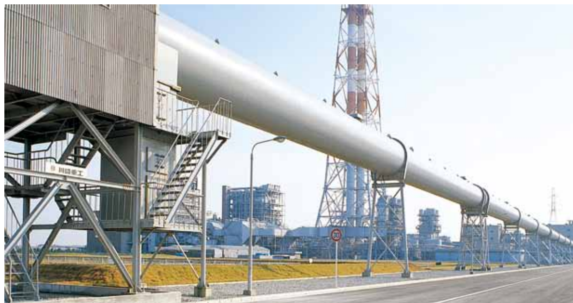
200 T/H belt conveyor (Tube gallery)
