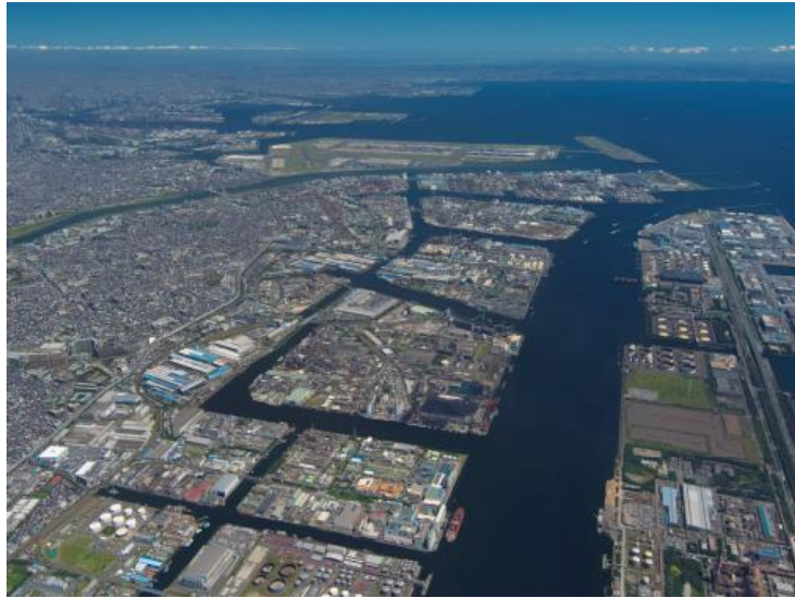
Air photograph of Resonac's Kawasaki Plant (the central part)
