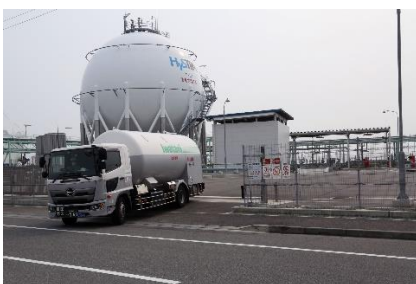
Hydrogen is transported from the LH2 Loading & Unloading Terminal
