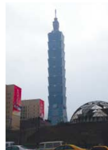
The world's tallest building, Taipei 101 (508 m).
