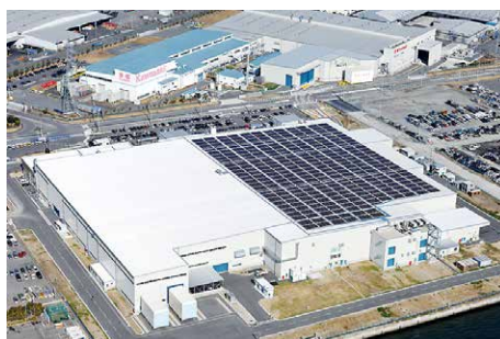
Figure 9: Nagoya Works 1: 750-kW power generation facility
