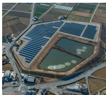
Figure 10: Kawasaki Trading Co., Ltd. Iwaoka Photovoltaic Power Generation Station: 1,505-kW power generation facility
