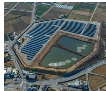
Figure 10: Kawasaki Trading Co., Ltd. Iwaoka Photovoltaic Power Generation Station: 1,505-kW power generation facility
