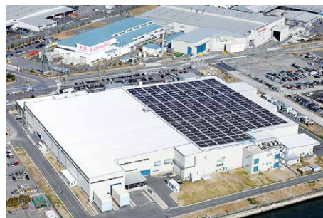
Figure 9: Nagoya Works 1: 750-kW power generation facility
