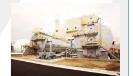
The biogas generation facility appearance of the fermentation tank
