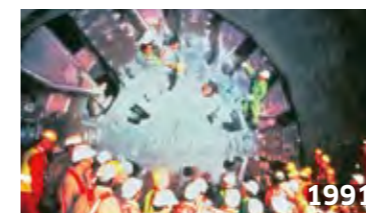
1991 Tunnel boring machines successfully complete work on the Eurotunnel
