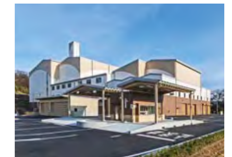
Incineration Plant of Matsusaka City
