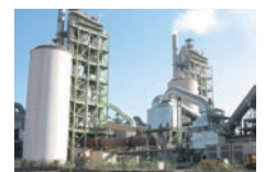
WHRPG in cement plant in Pakistan
