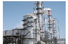
Flue gas Desulfurization System (Saudi Arabia)
