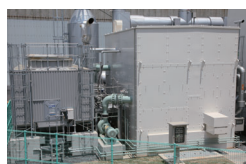
Binary power generation system
