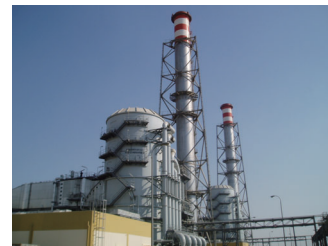
Flue gas de-SO x system (Saudi Arabia)
