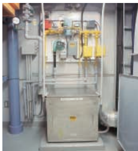
Burner control equipment
