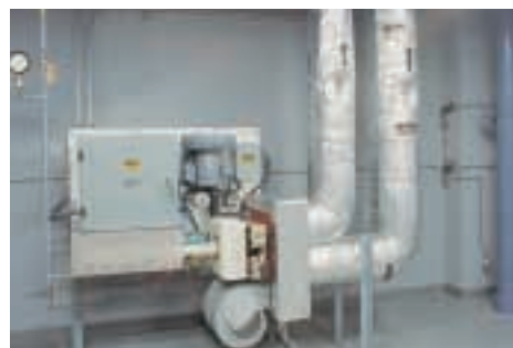
Mock smoke generation equipment
