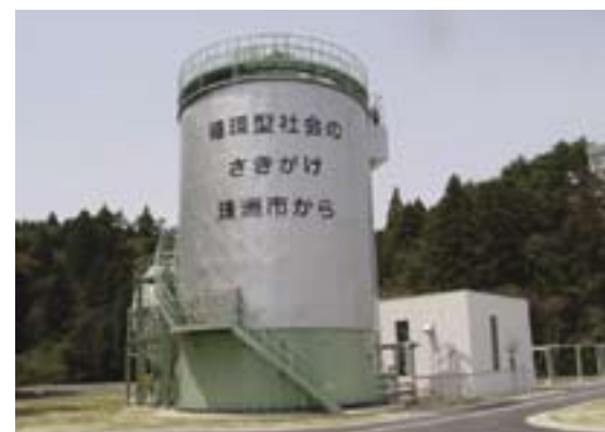
Methane fermentation system for biomass resources
