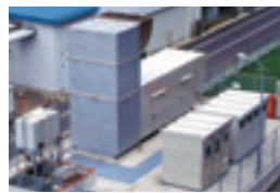
Emergency gas turbine generator
