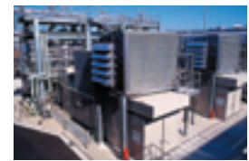
Gas turbine cogeneration system
