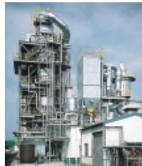
Internal circulation fluidized bed-type incineration system
