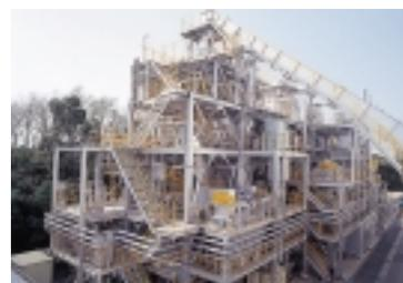
Fluidized bed-type gasifying-melting system
