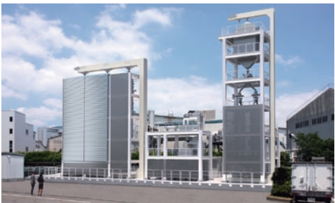
New DAC and PCC demonstration facilities
