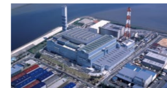
1997 Completed municipal waste incineration facilities for the Shin-Nanyo Plant in Nagoya City
