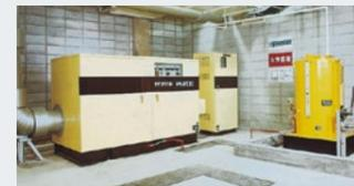
1976 Developed the *Kawasaki GPS200*, the first Japan-made gas turbine generator
