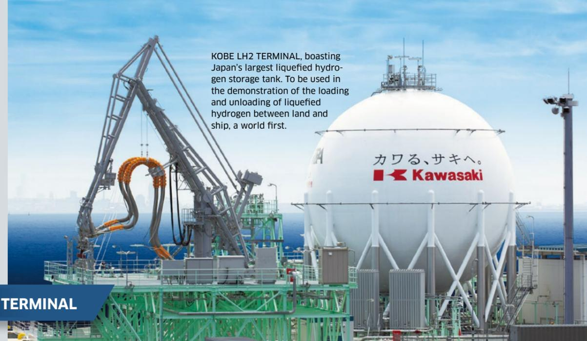
KOBE LH2 TERMINAL, boasting Japan's largest liquefied hydrogen storage tank. To be used in the demonstration of the loading and unloading of liquefied hydrogen between land and ship, a world first.
