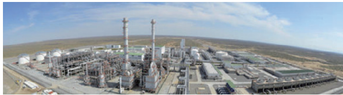
Gas-to-gasoline (GTG) plant
