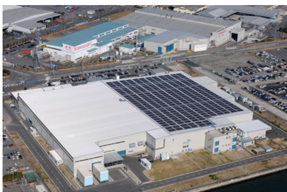
Nagoya Works 1: 750-kW power generation facility
