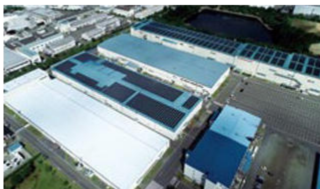
Seishin Works: 1,444-kW power generation facility
