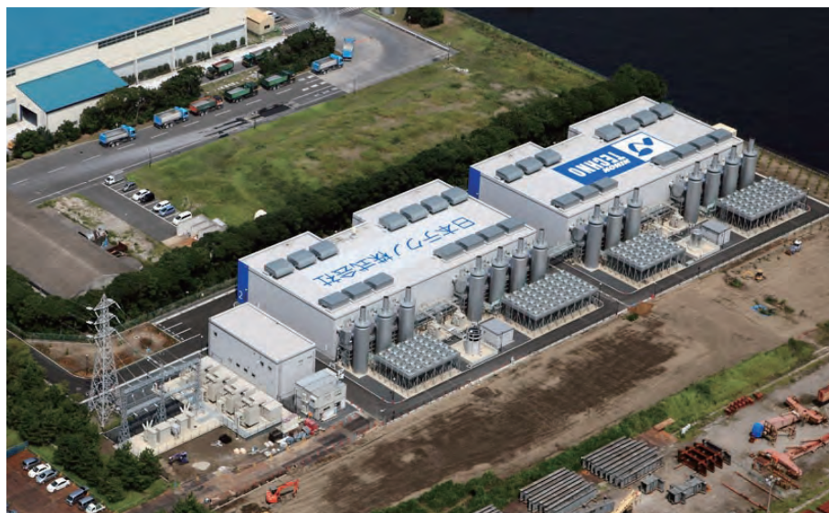
Fig. 8 110 MW class power station delivered to Nihon Techno Co., Ltd.
