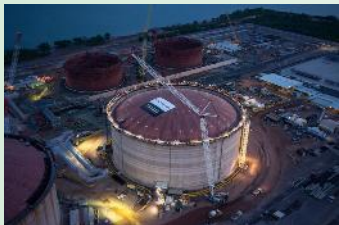
liquefied natural gas (LNG) tanks
