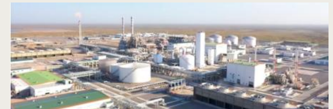
Gas-to-Gasoline (GTG) Plant Constructed by KHI in Turkmenistan Production Capacity: 600,000 tons/year
