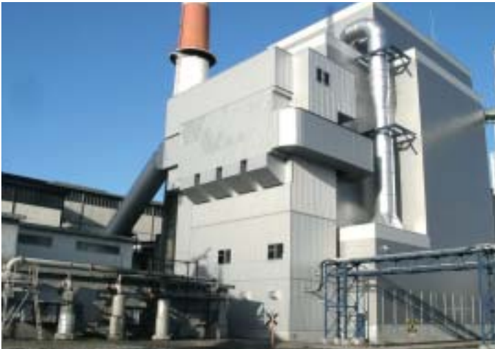
Coal-fired power plant for internal power requirements at the Memuro plant of Nippon Beet Sugar Manufacturing Co., Ltd.
