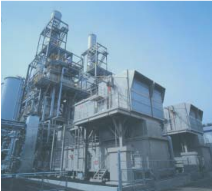
Combined cycle power plant utilizing L20A gas turbine generators for the Chiba Mihama Power Generation Project
