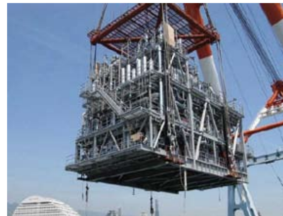
Single lifted Gas Compression Module for KNOG
