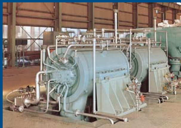
Tandem arranged steam turbine driven compressors for ammonia gas service, Ube Ammonia (Japan)
