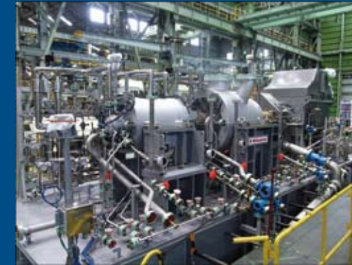
Motor driven compressor for FPSO, PTSC (Vietnam)
