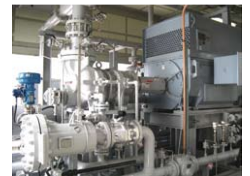
Shop Fuel gas compressor for GT drives
