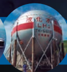
Long term storage of liquefied hydrogen
