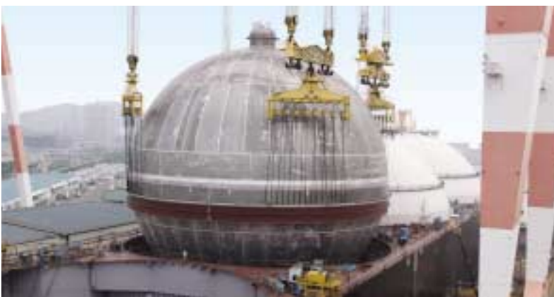
The spherical tank is slowly lowered into the skirt.
