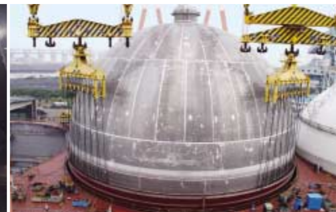
The tank is now in place.
