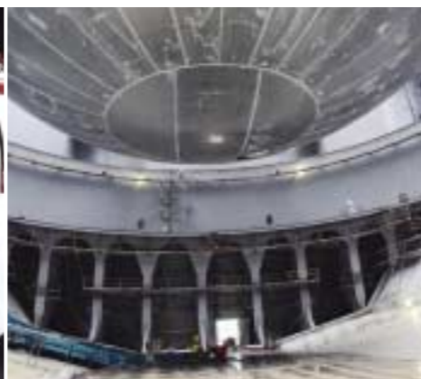
The tank is steadily lowered. The bottom of the skirt comes into view.
