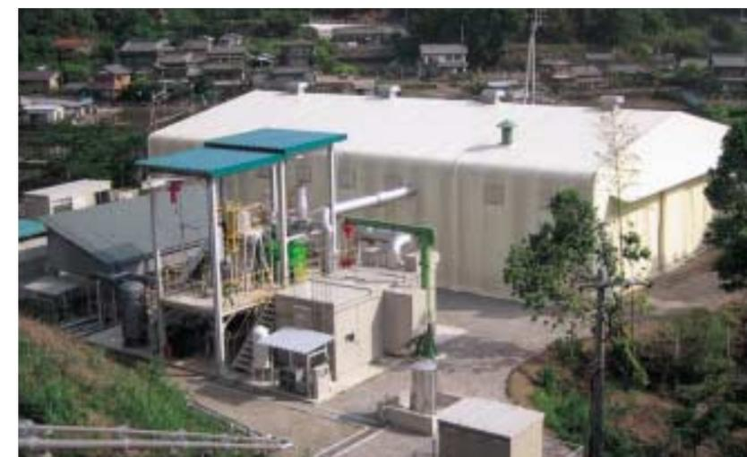
is directed to the gas turbine combustor while maintaining the same temperature and pressure. This allows for effective use of the tar which would normally have to be removed with water in conventional systems. Thanks to these features, it's three times more efficient for generating power than direct-combustion biomass power generation systems and can be applied to small-scale woody biomass systems.
