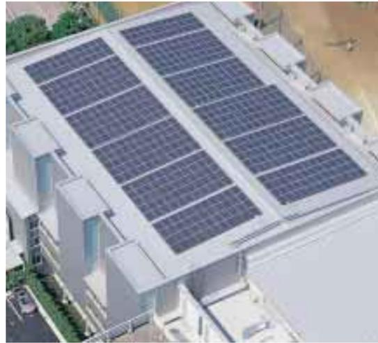
Solar battery modules installed on Yachiyo Shoin Gymnasium No. 1
