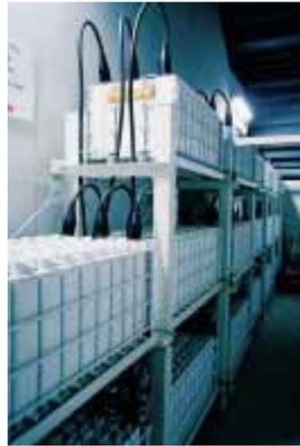
Gigacell installed in the basement of Gymnasium No. 1
