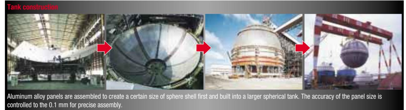
Aluminum alloy panels are assembled to create a certain size of sphere shell first and built into a larger spherical tank. The accuracy of the panel size is controlled to the 0.1 mm for precise assembly.
