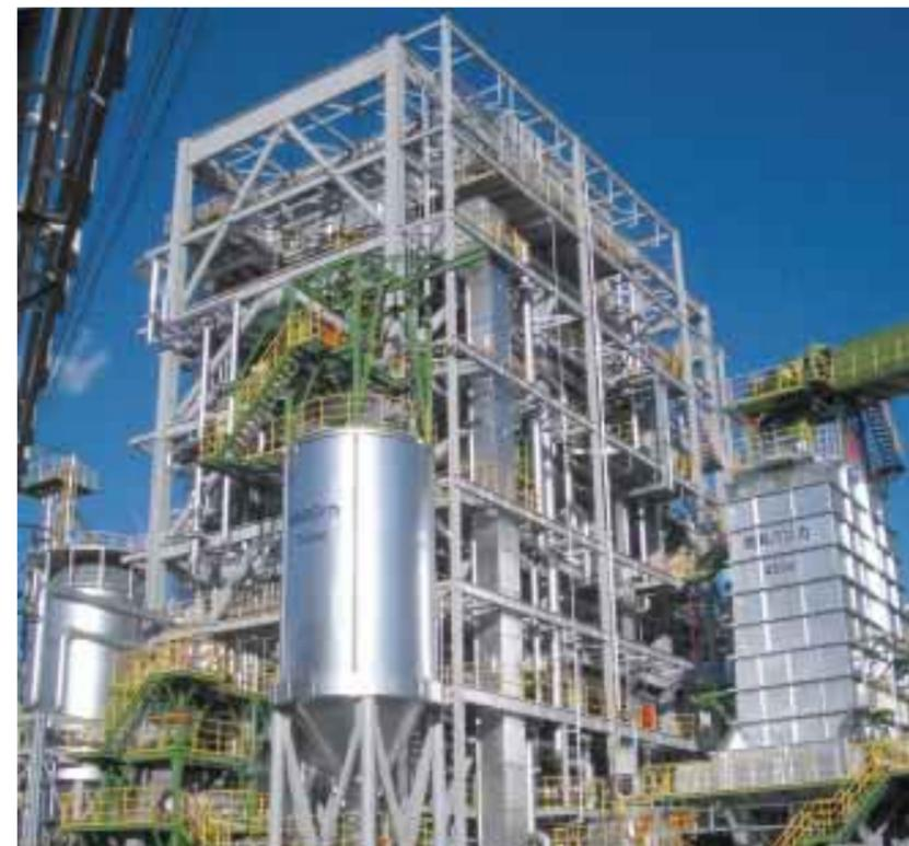
This steam, combined with steam from another boiler installed earlier at the plant, feeds the power-generating turbine and is used for drying paper and other papermaking processes at the mill. The introduction of an axial exhaust turbine contributed to lowering the height of the turbine building.
