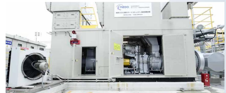
At the heart of the co-generation system on Kobe's Port Island (photo on page 4) is this hydrogen gas turbine, which drives the power generator, and using waste heat, operates the boiler.
