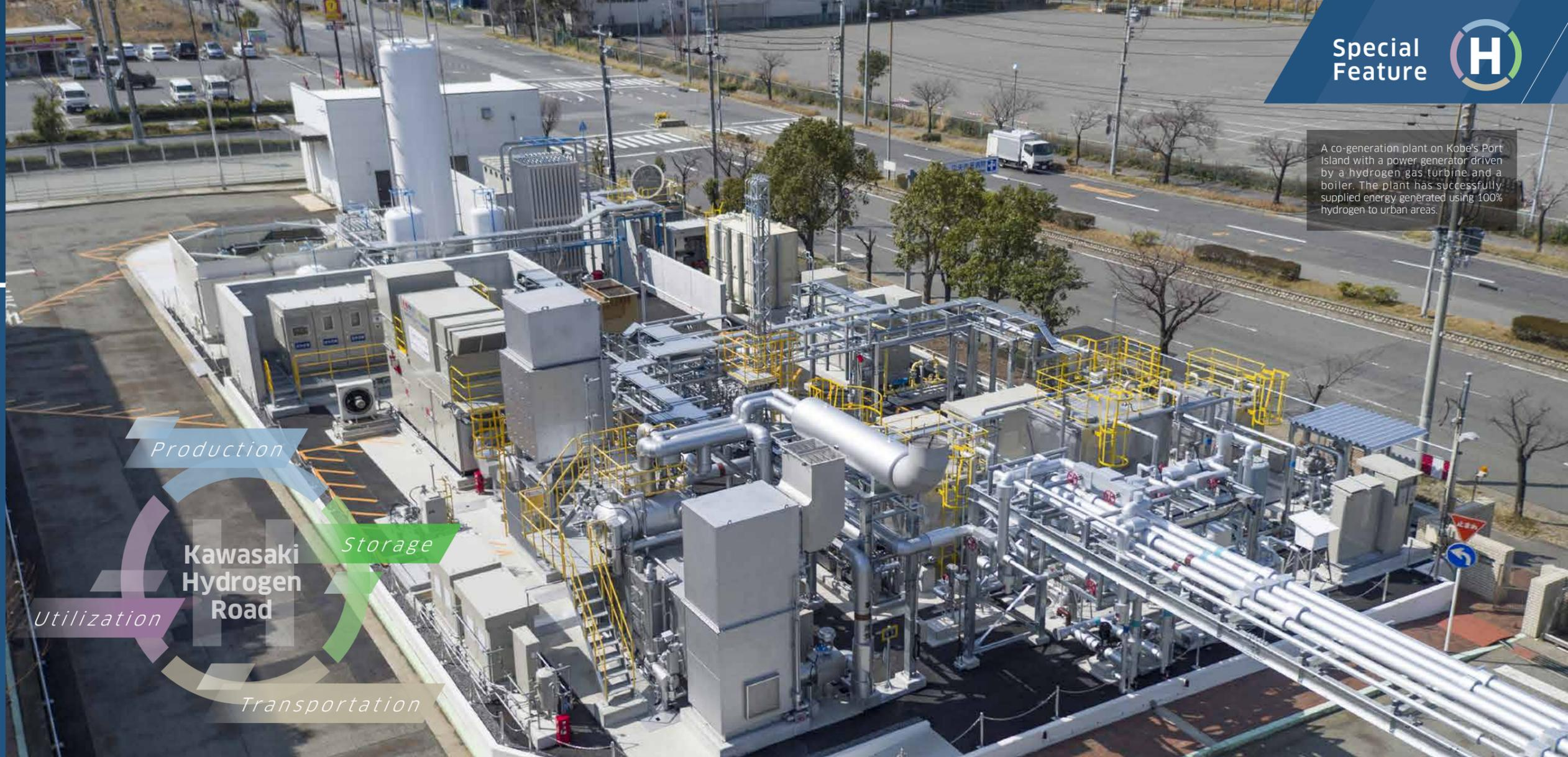
A co-generation plant on Kobe's Port Island with a power generator driven by a hydrogen gas turbine and a boiler. The plant has successfully supplied energy generated using 100% hydrogen to urban areas.
