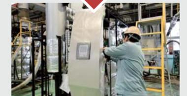
Finally, a cover casing is installed. The door's front panel is equipped with a controller used for remote monitoring of the boiler via communication lines.
