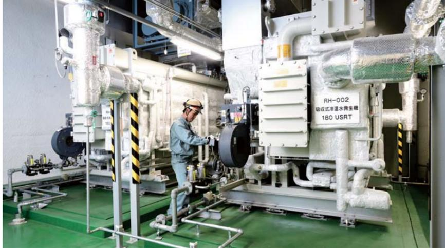
The Efficio absorption chiller-heater in operation at Osaka Medical College Hospital. Two Efficio units cool and heat the entire Surgery Building. With dual lines—one dedicated to cooling and another to heating—the hospital can control both temperature and humidity to optimize the surgical environment of each operating room according to its needs.
