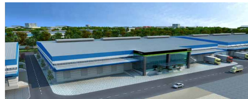
Image of new plant.
