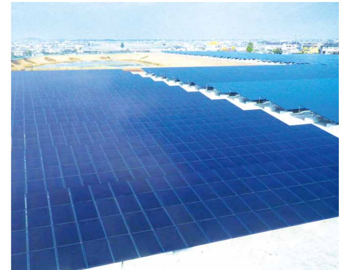
Location: Former Iwaoka landfill Capacity: 1,500 kW Start of operation: March 2014
