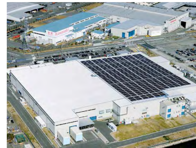
Location: First Nagoya Plant of Kawasaki Heavy Industries Capacity: 750 kW Start of operation: January 2011
