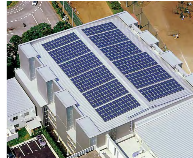
Location: First Gymnasium in Yachiyoshoin Gakuen School Capacity: 100 kW + GIGACELL Start of operation: July 2005
