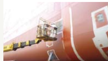
Welding inspection using an aerial work platform
