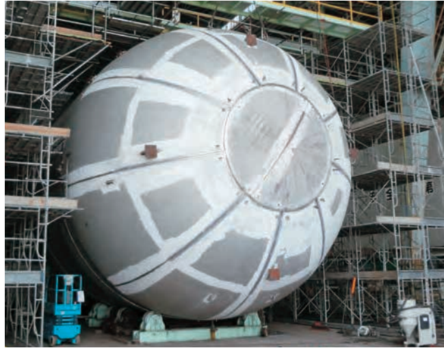
Fig.5 Trial manufacture of aboveground LH 2 tank
