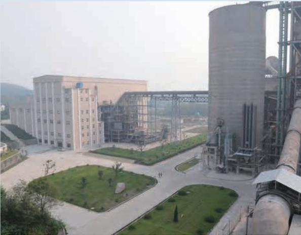
*The CKK System is a new waste incineration system jointly developed by Kawasaki and the Anhui Conch Group, its joint venture partner in China. This innovative system achieves hygienic waste treatment at low cost, and also makes effective use of the energy and ash content of waste as fuel and raw material for cement production. Orders for the CKK System are steadily increasing in China.*
