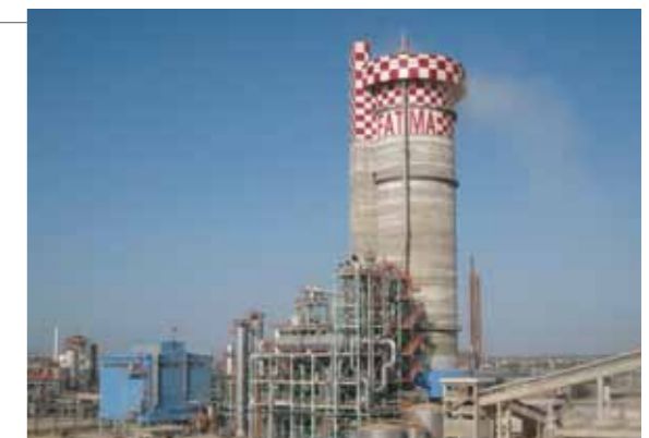
Urea manufacturing facility
